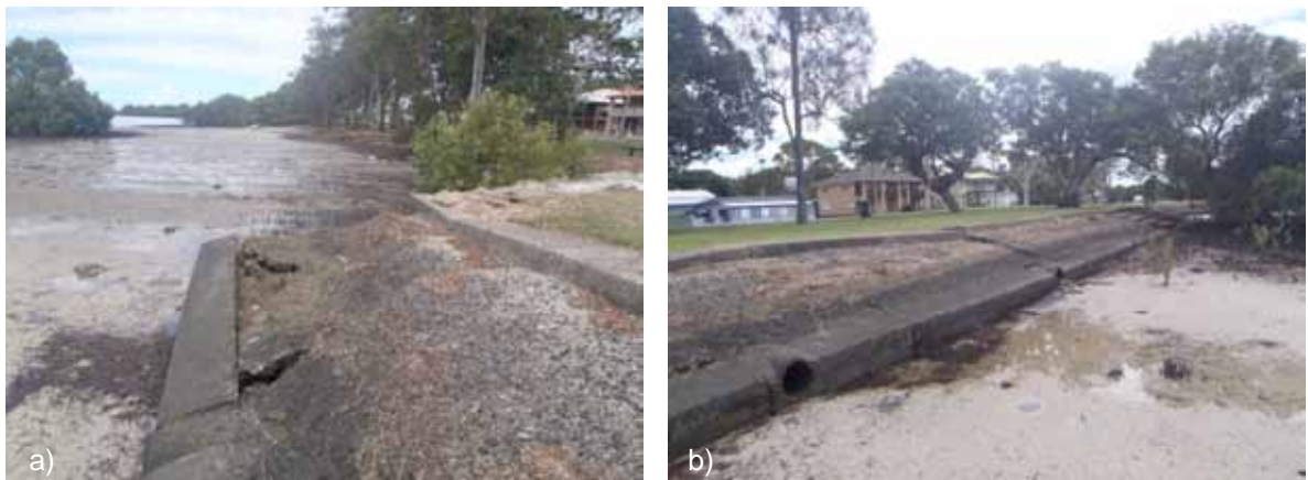
Figure 6-4 Sloping Concrete Seawall Damage Opposite Willmer Road
