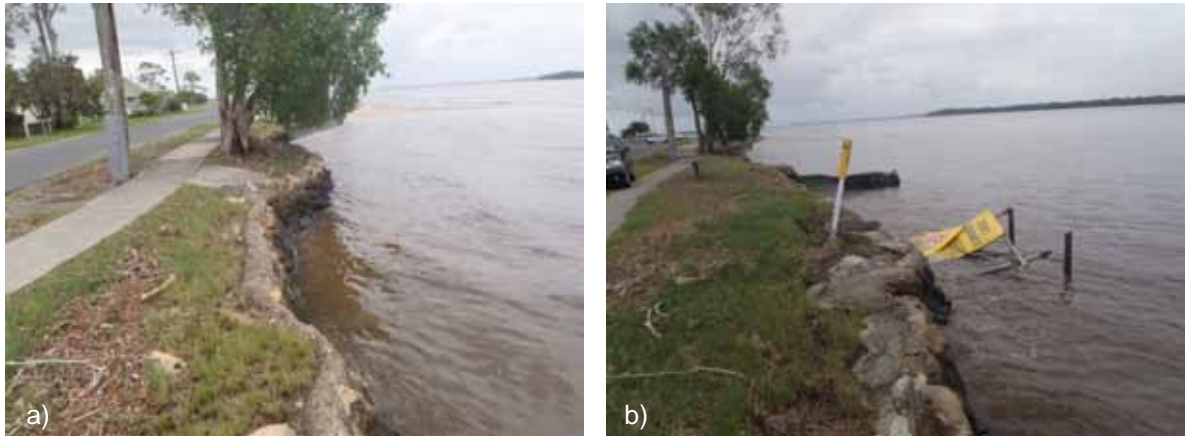
Figure 6-3 Unapproved Seawall Opposite Second Ave: a) Narrow Section between Pathway and Seawall Crest; b) Sinking Damage following ex-TC Oswald (January 2013)
