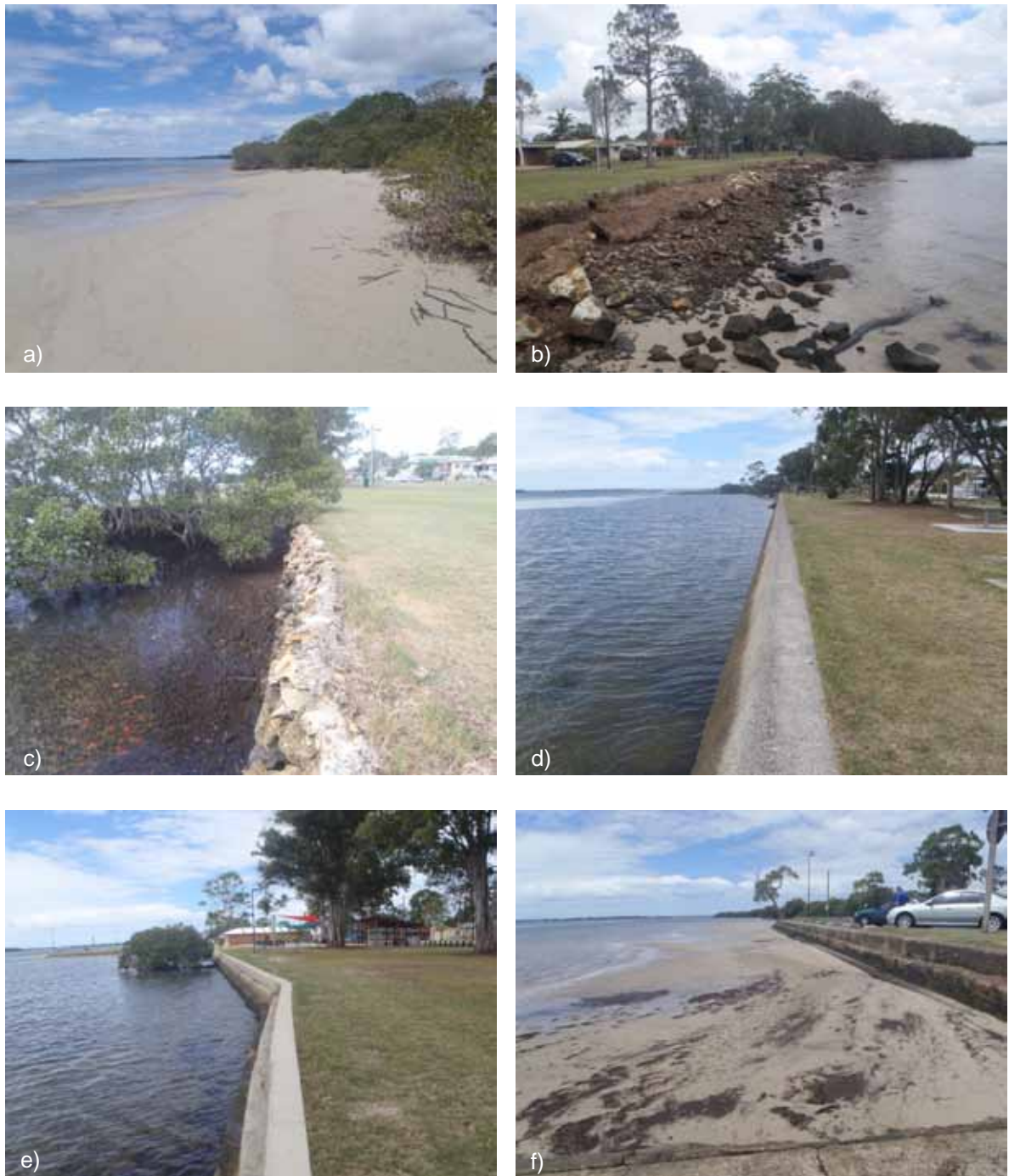
Figure 6-2 Example Shoreline Condition throughout Toorbul Study Area: a) Sandy Shore with Mangrove; b) Loose Rock and Erosion Scarp; c) Stone and Concrete Seawall; d) Stepped Seawall with Shotcrete Repair; e) Stepped Seawall; f) Stepped Seawall with Sand Accumulation at Boat Ramp
