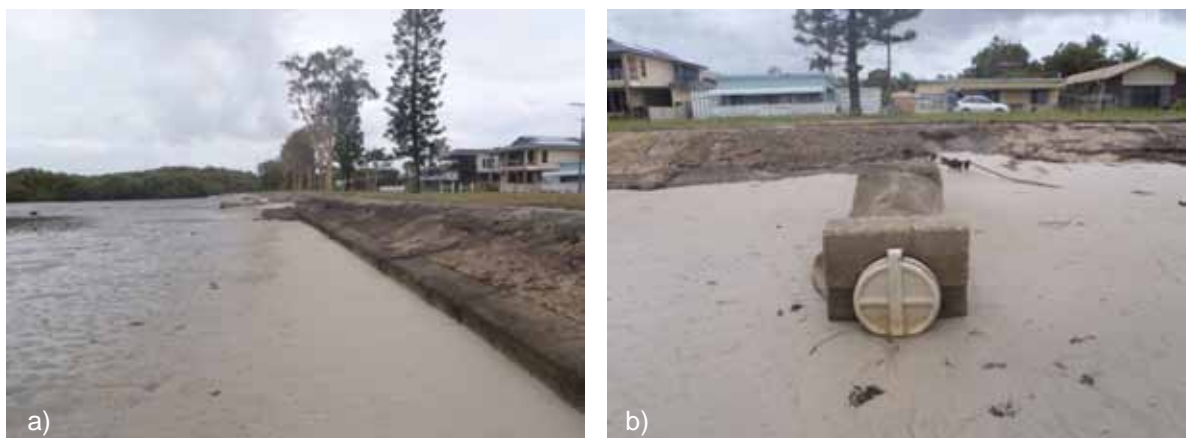
Figure 4-1 Example Shoreline Condition throughout Godwin Beach Study Area: a) Sloped Concrete Seawall; b) Stormwater Drainage Pipe
