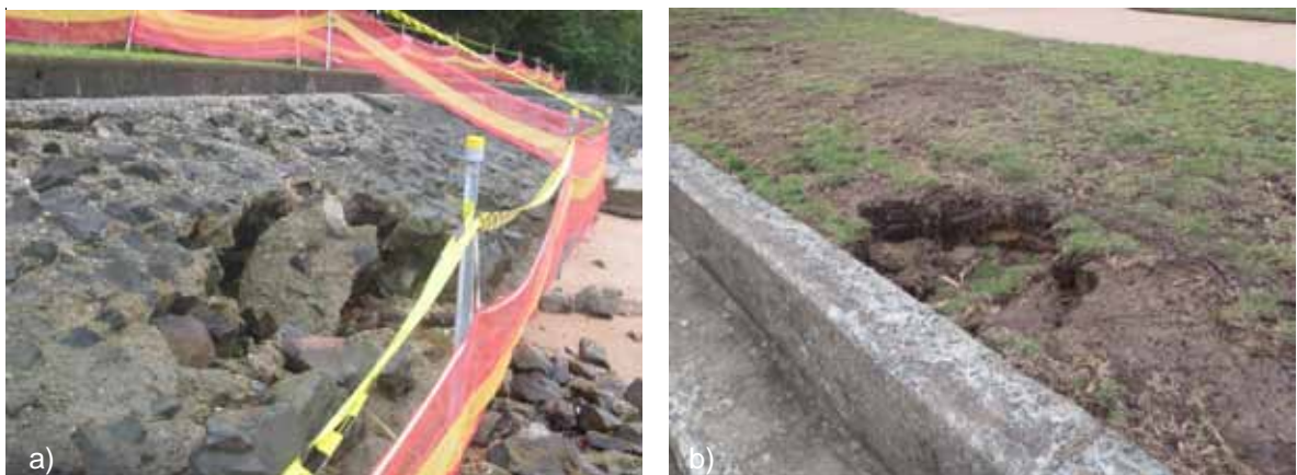
Figure 2-3 Seawall Damage January 2013: a) Stone Pitched Seawall Failure (prior to Shotcrete Repair); b) Sink Hole behind Stepped Seawall
