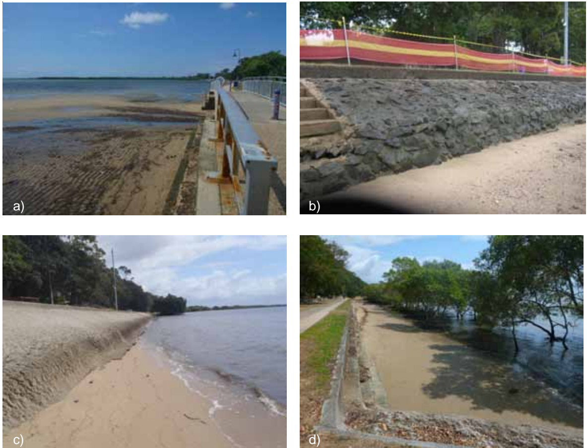
Figure 2-2 Example Shoreline Condition throughout Deception Bay Study Area: a) Stepped Concrete; b) Stone Pitched; c) Stone Pitched with Shotcrete Repair; d) Stepped Concrete with Mangrove Buffer
