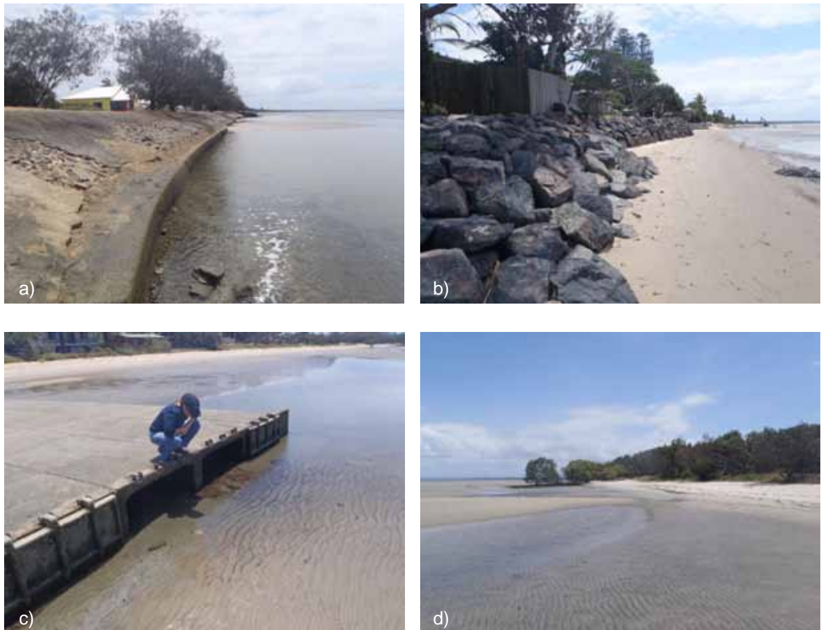
Figure 3-2 Example Shoreline Condition throughout Beachmere Study Area: a) Stone Pitched Seawall with Shotcrete Repair; b) Loosely Placed (foreground) and Tightly Packed (background) Rock Seawalls; c) Storm Water Culvert and Low Vegetation Shoreline (background); d) Beach with Dense Coastal Vegetation
