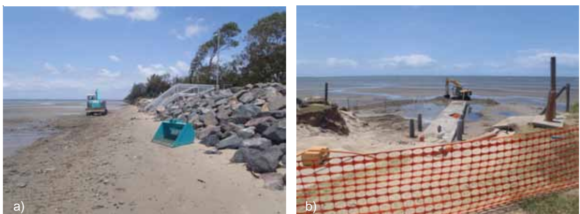
Figure 3-3 Recent Upgrades to Council Controlled Areas: a) Beachmere Activity Centre Rubble Seawall and Beach Access; b) Albert and Myrtle Lehman Park Culvert Upgrade
