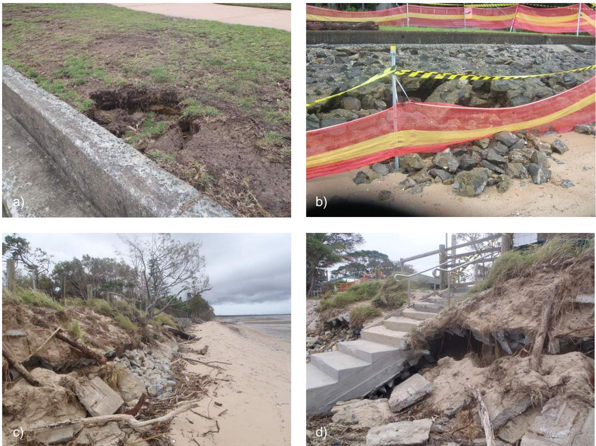
**Figure 5-16 Recently Observed Shoreline Erosion: (a) Sink Hole and (b) Seawall Failure at Captain Cook Parade, Deception Bay; (c) Exposed Shoreline Fill and (d) Closed Beach Access at L & M Lehman Park, Beachmere**
