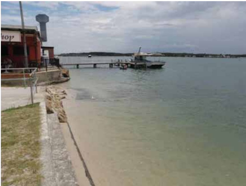
Photo Plate 6-4 Jetty facilities
