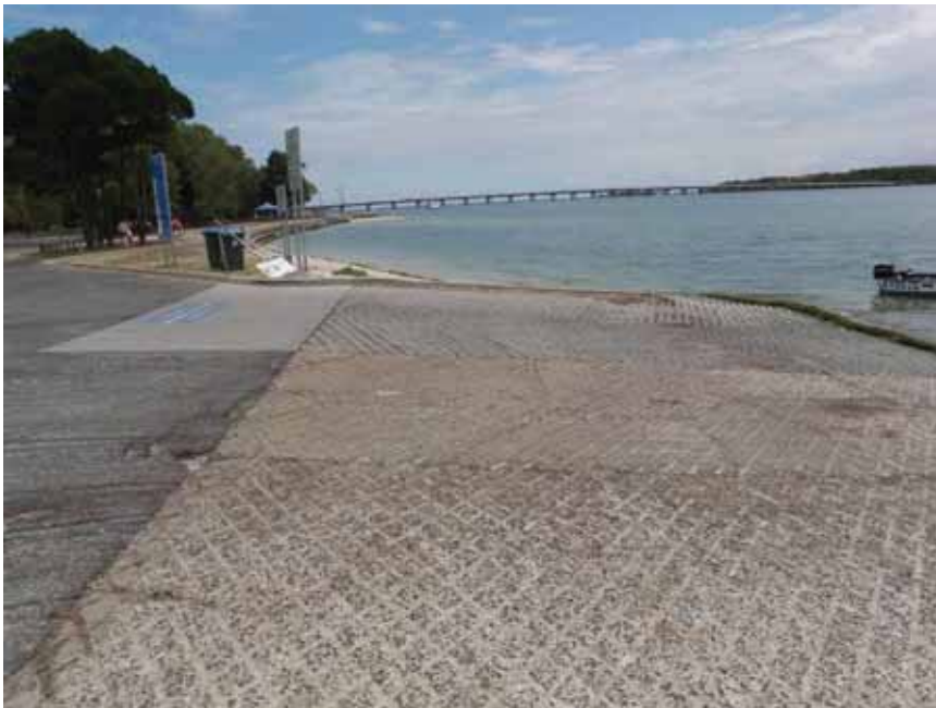
Photo Plate 6-2 Boat ramp
