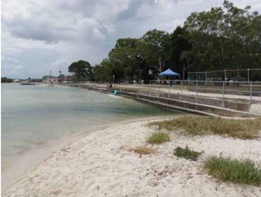
Photo Plate 6-1 Drainage canal culvert outlet south of boat ramp
