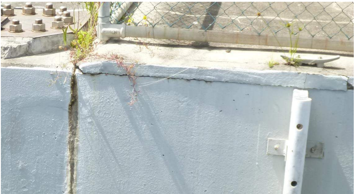
Figure 4-11: Lock S Wall (Lock Island) 20/01/16 – Cracking and growth on lock island topping adjacent to cleats and other fixings
