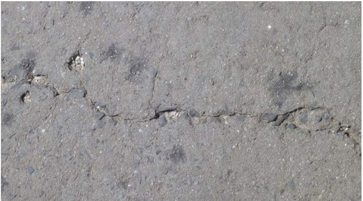
Figure 5-1: Weir Walkway 20/01/16 – Cracking of top of walkway deck at weir wall support
