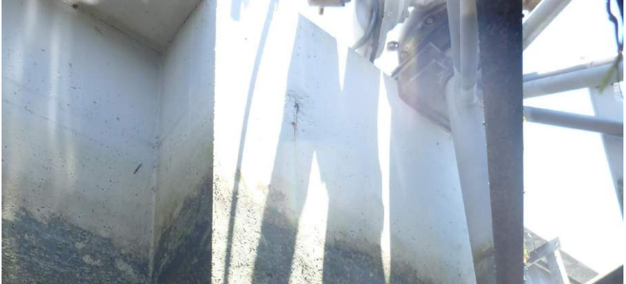
Figure 4-3: Lock Island SW Gate Recess 20/01/16 – Poor compaction and very low/zero cover on gate attachment wall, corrosion staining visible
