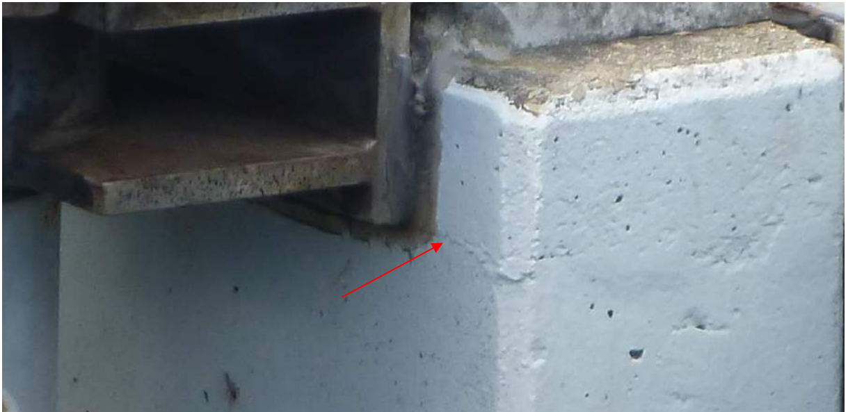
Figure 4-5: Lock SW Gate Recess 20/01/16 – Crack at top to the north of gate hinge connection (identified by red arrow)
