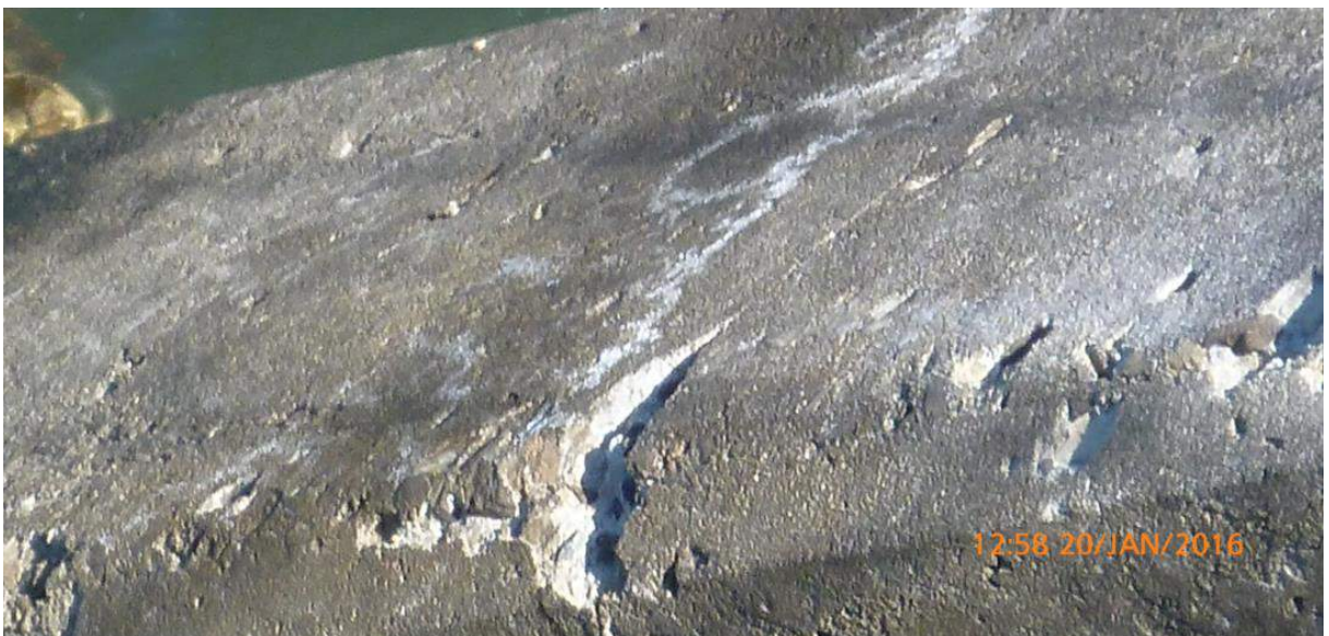
Figure 5-2: South Weir Wall 20/01/16 – Impact damage to upstream side
