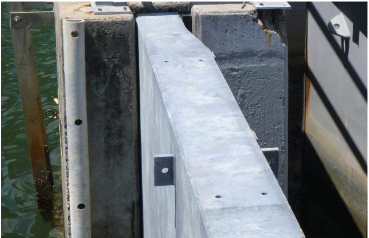
Figure 4-10: Lock SE Gate Recess 20/01/16 – Outer ladder lower connection appears missing
