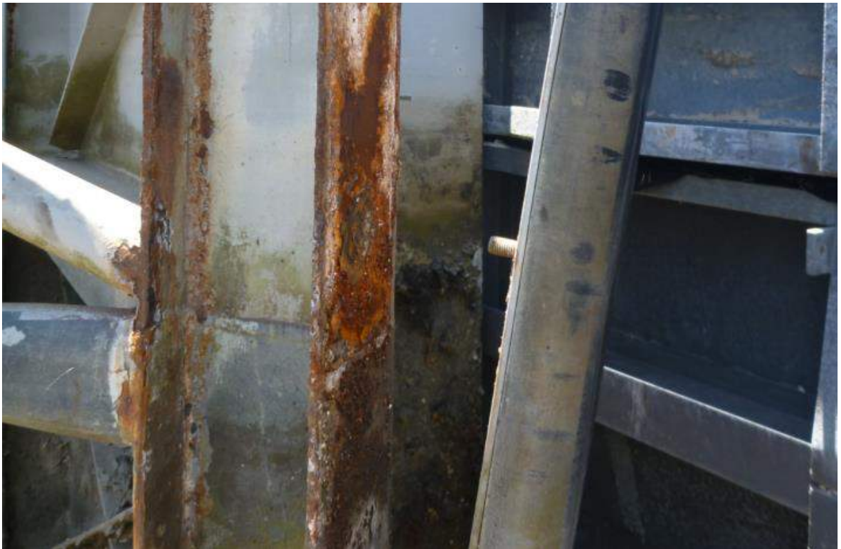
Figure 4-6: Lock NE Gate 20/01/16 – Gate to Gate seal pulled back to reveal extent of corrosion on vertical parallel flange channel member – ultrasonic thickness measurements identified negligible section loss to steel members
