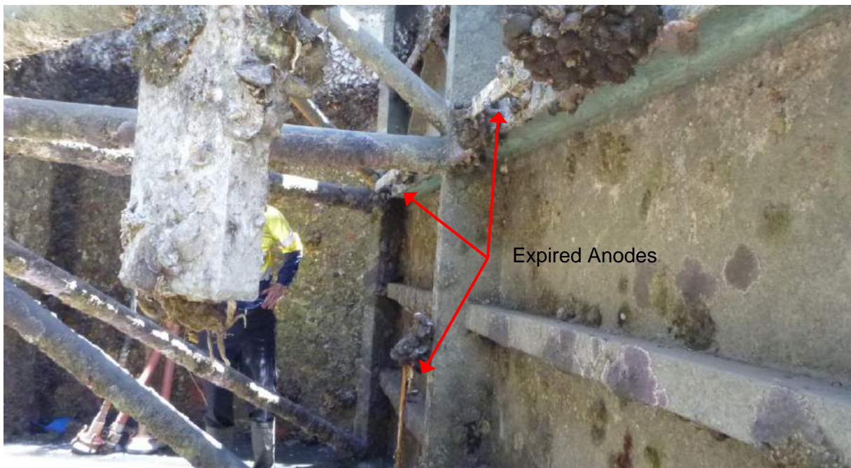
Figure 4-7: Lock NW Gate 20/01/16 – Inside face, 3 anodes (2 vertical, 1 horizontal – identified with red arrows) completely expired
