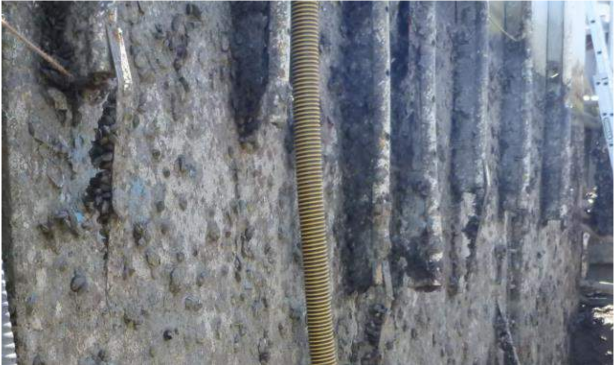
Figure 4-8: Lock N Wall Fenders 20/01/16 – Lower fender connections missing and failed
