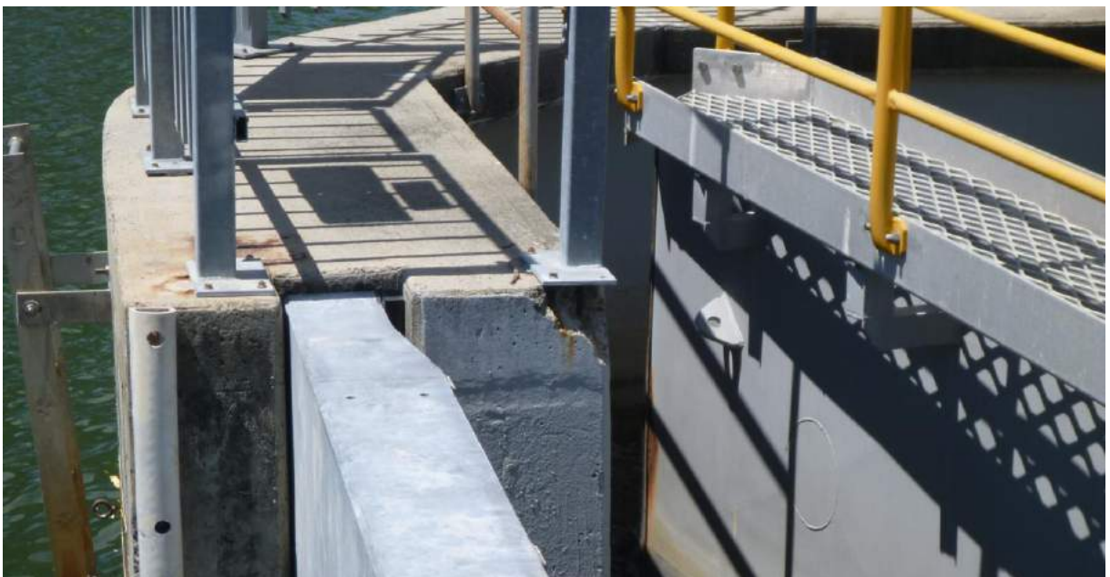
Figure 4-2: Lock Island Walkway SE Gate Recess 20/01/16 – Spall beneath handrail stanchion
