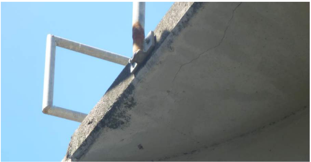
Figure 4-4: Lock SW Gate Recess 20/01/16 – Crack on walkway cantilever slab section
