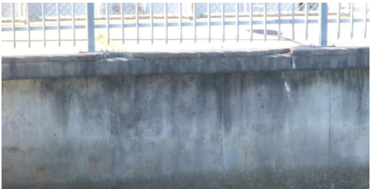
Figure 4-12: Lock Island (view from weir) 20/01/16 – cracking and spalling to edge of lock island topping slab adjacent to fencing fixings
