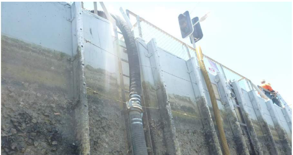
Figure 4-9: Lock N Wall Ladders 20/01/16 – Ladders fouled by stainless steel wire rope between fenders
