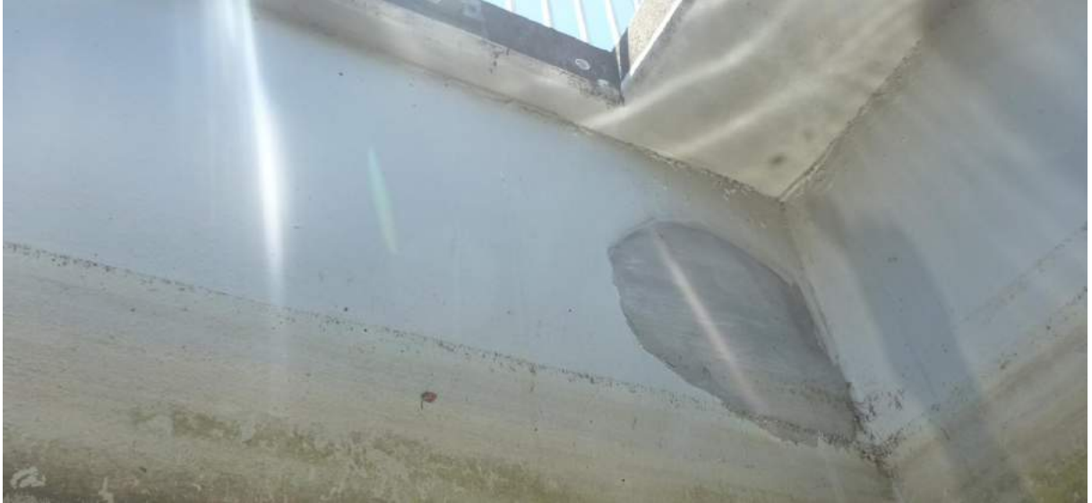
Figure 4-1: Lock SE Gate Recess 20/01/16 – Spall repair starting to fail at west end inner south wall of SE Recess
