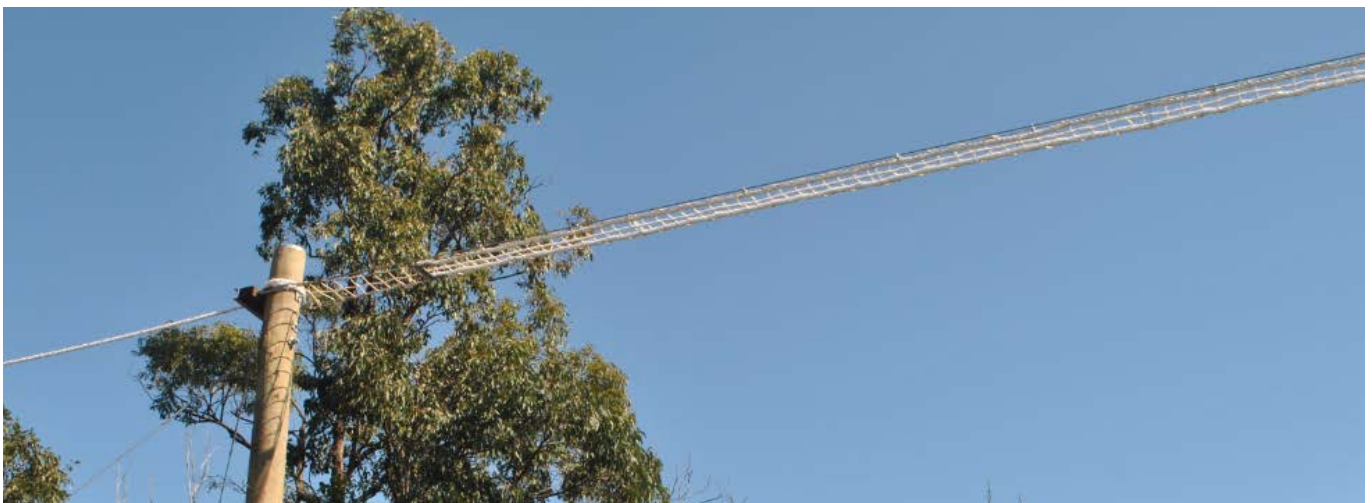
Fauna rope bridge installed at Old North Road, Warner in 2016.
