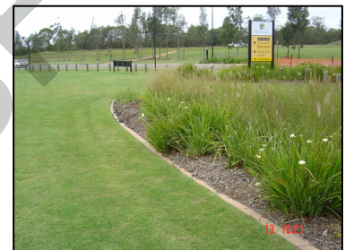
Built edges must be installed at the grass mulch interfaces in parks and commercial and retail centres (North Lakes Town Park)
