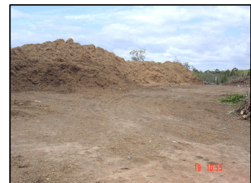
Cleared vegetation is volume reduced by chipping or grinding and stockpiled on site (Dakabin Rubbish Tip)
