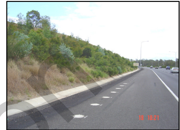
Hydro-mulching is used for erosion control on batters and slopes unable to be mown with conventional equipment (Bruce Highway, Murrumba Downs)
