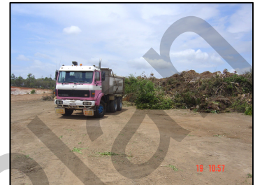
Rubbish located on proposed crown land is to be removed and appropriately disposed of at a landfill site (Dakabin Rubbish Tip)
