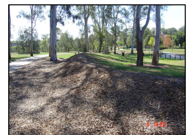
Mounding is designed and constructed with regard for maximum slope requirements (Wyllie Park, Petrie)
