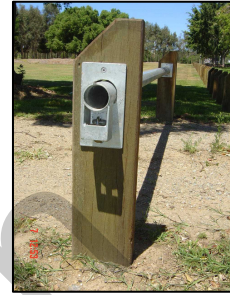
Council specified removable access sliprail (Pine Rivers Park, Strathpine)
