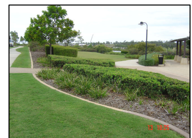
Edging must be able to sustain the movement of tractor mowers (North Lakes Town Park)
