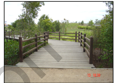
Boardwalks are designed and constructed using sound, robust and durable practices (North Lakes Town Park)
