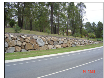
Where vegetative cover is not achievable on extreme slopes, retaining walls are required. (Lilley Road, Cashmere)
