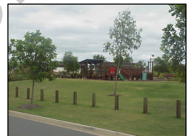
Vehicle exclusion devices must be provided along road frontages (Settlers Park, North Lakes)
