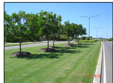
In median strips three (3) metres or wider trees may be located centrally or staggered provided such accords with traffic engineering visibility requirements. (Discovery Drive, North Lakes)
