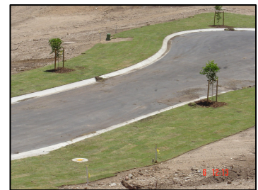
Turf is to be laid with edges butted up and is to be rolled into topsoil after watering (Eatons Rise Estate, Eatons Hill)
