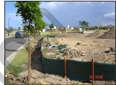
Erosion and sediment controls are constructed prior to commencement of any clearing works (Glenrock Parade, North Lakes)
