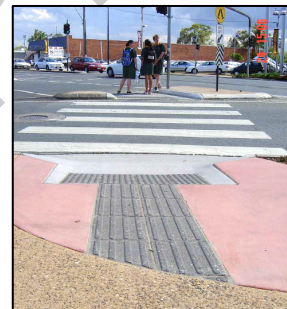
Tactile surface indicators are provided to aid users with vision impairment (Cnr Learmonth Street and Gympie Road, Strathpine)
