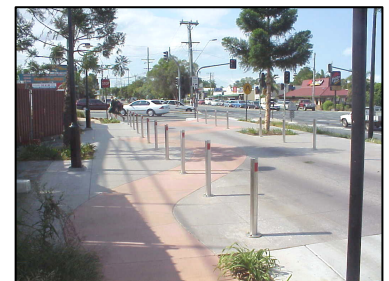
New surfacing should provide ease of movement and complies with AS148 Design for Access and Mobility (Gympie Road, Strathpine)
