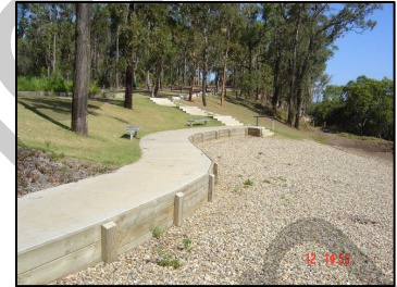
Retaining walls are designed and constructed for function, durability and maintenance access (Old Northern Road, Albany Creek and Acacia Park, Murrumba Downs)
