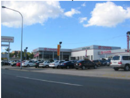
Image 9 - Unacceptable Incoherent layout and access arrangement with no landscaping to soften and enhance the built form. Unattractive built form and roofscape that does not provide visual relief or provide visual interest for passers by.
