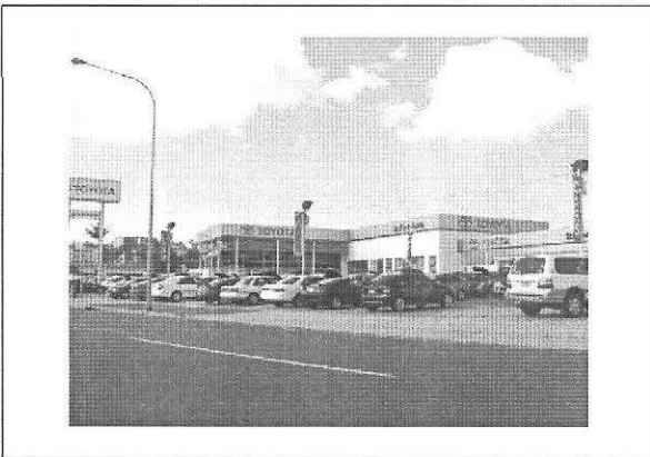
Image 9 - Unacceptable Incoherent layout and access arrangement with no landscaping to soften and enhance the built form. Unattractive built form and roofscape that does not provide visual relief or provide visual interest for passers by.
