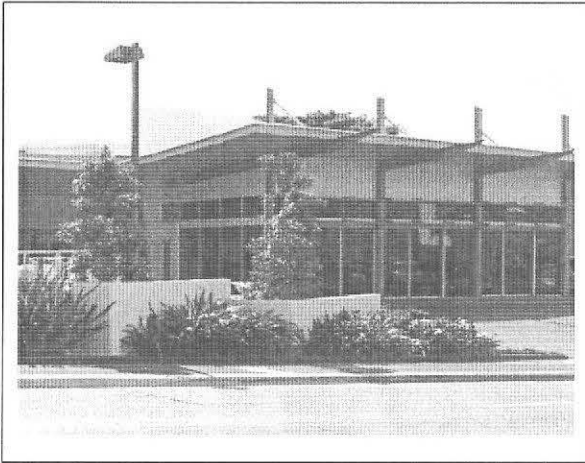
Image 7 - Acceptable Generally frame entry areas to sites.
