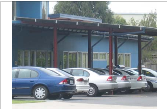
Image 7 – Acceptable Surface car parking may include shade structures within selected areas of the car park.
