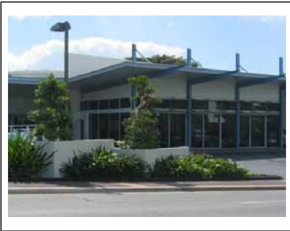
Image 7 - Acceptable Generally frame entry areas to sites.
