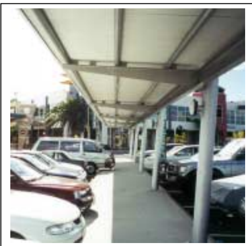
Image 59 – Acceptable. Wheel stops are to be used to ensure pedestrian movement is not compromised. Acceptable shade structures over pedestrian routes in car parks.
