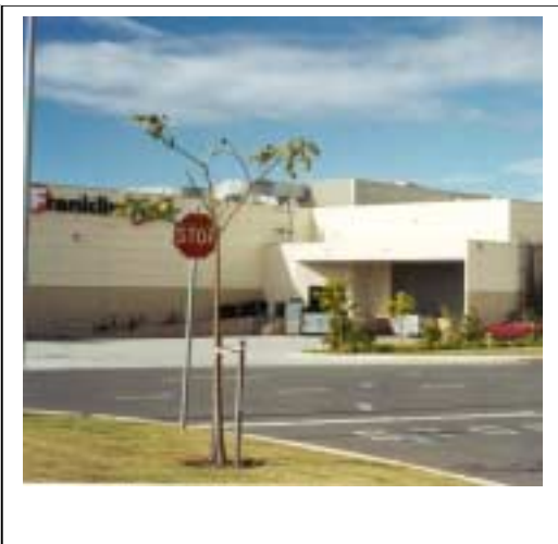
Image 15 - Unacceptable. Service areas, loading bays and refuse areas will be screened.
