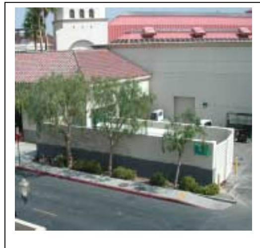
Image 16 - Acceptable. Appropriate screening of service area.
