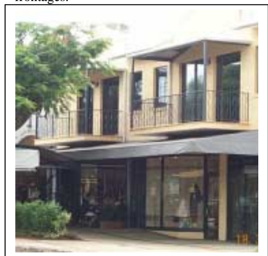
Image 24 - Acceptable. Windows at upper levels provide for viewing of external areas.
