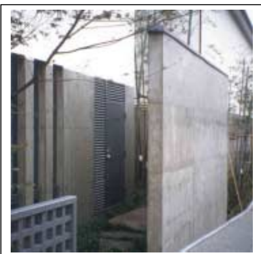
Image 17 - Acceptable. Appropriate screening of service area where CPTED principles are not compromised.
