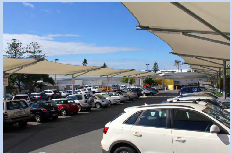
(Coolum) Car parking area at rear.
