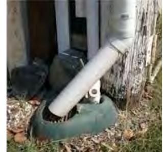
The illegal connection of stormwater infrastructure to the sewerage system significantly increases the volume of water in the sewerage systems, which can result in the capacity of the network being exceeded. This can cause the network to overflow, resulting in environmental harm and creating risks to human health. Major capital expenditure is also required to mitigate this through the construction of larger pipes, pump stations and treatment plants.
