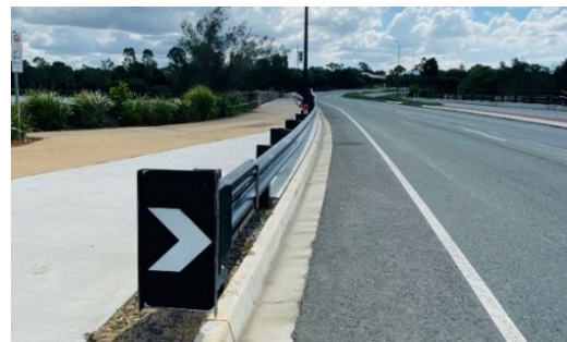
Figure 8 - Example of guardrail (Discovery Drive, Northlakes)
