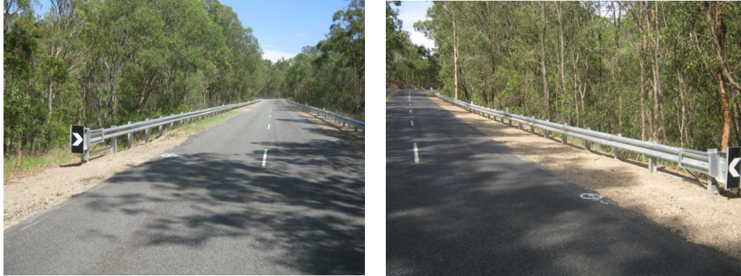
Figure 35 - Examples of Recently Renewed Guardrails
