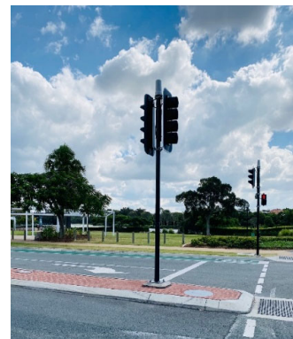
Figure 22 - Traffic Signal (Memorial Drive, Northlakes)
