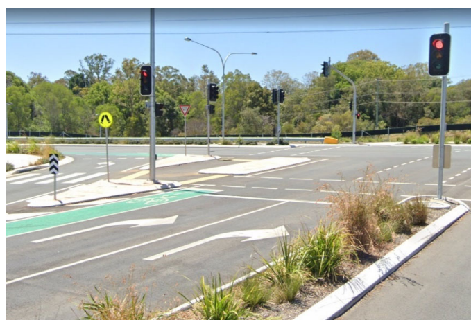
Figure 1 Typical road furniture including traffic islands, signals, cycleways, kerb and channel, guardrails and signage (Russet Burbank Pde, Warner)
