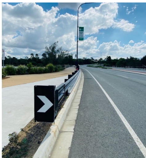
Figure 26 - Example of guardrail (Discovery Drive, Northlakes)
