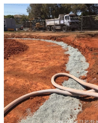
Figure 23 - Example of subsoil drainage being installed
