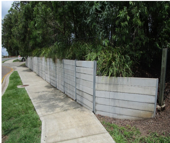
Figure 21 - Sheaves Road piled wall
