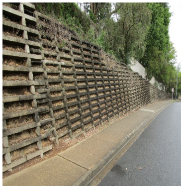
Figure 1 - Albany Forest Drive concrete crib wall
