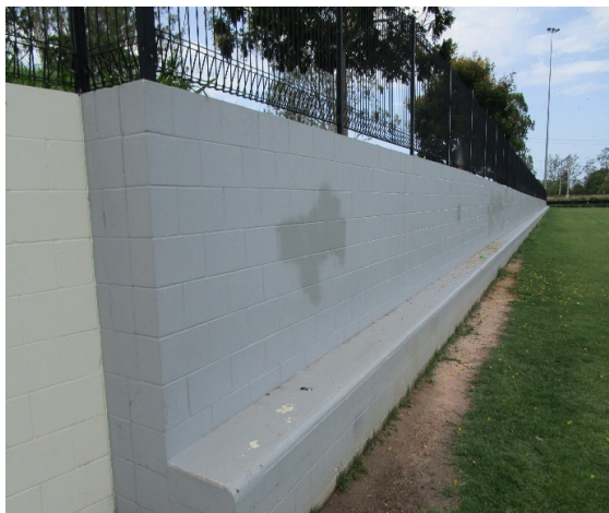
Figure 19 - Mathieson Park cantilevered wall
