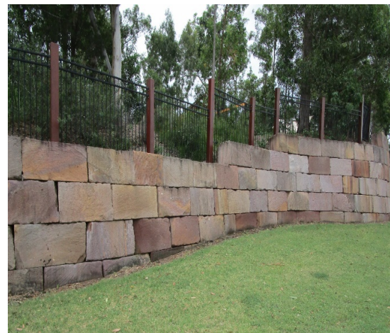
Figure 20 - Stoneridge Boulevard Park gravity wall
