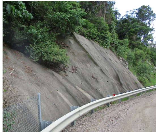
Figure 22 - Goat Track Road anchored wall
