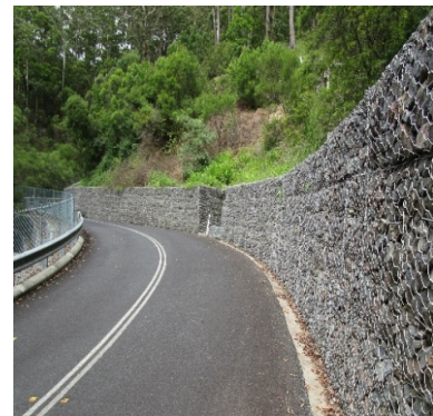
Figure 3 - Bellthorpe Range Road gabion rock wall
