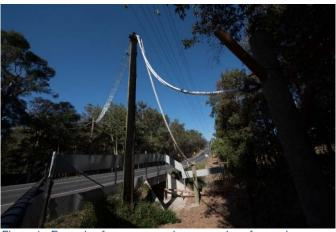
Figure 1 - Example of overpass, underpass and a refuge pole
