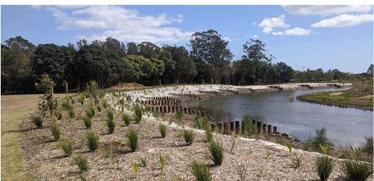
Figure 1 - Example of recently constructed bank stabilisation works at Pine Rivers Park, South Pine River
