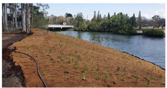
Figure 24 - the site of an erosion scarp at Wylie Park after bank stabilisation works
