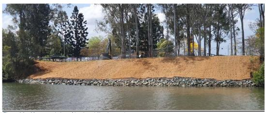
Figure 26 - After completion of bank stabilisation works
