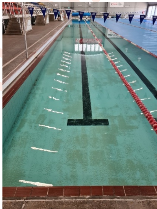
Figure 1: Image of 50m Pool Deterioration
