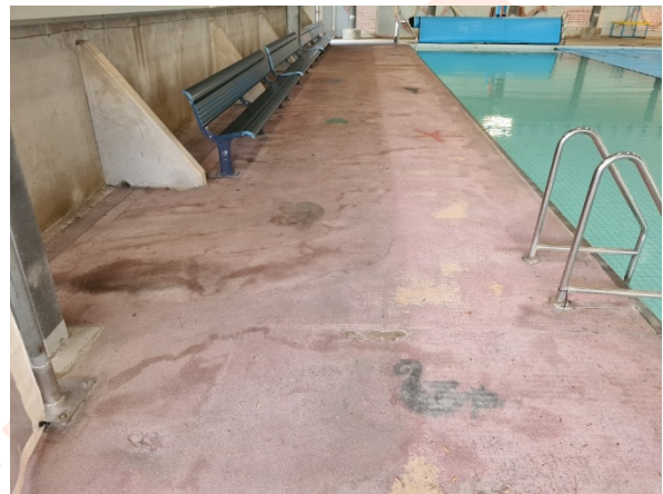
Figure 3: Image of Deteriorated Artwork (18.3m Pool)
