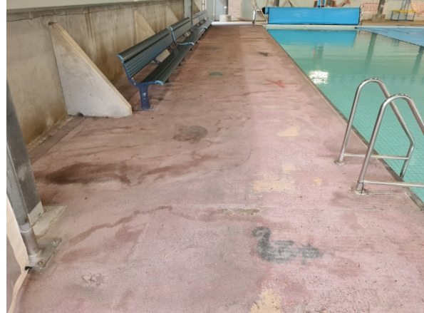
Figure 3: Image of Deteriorated Artwork (18.3m Pool)
