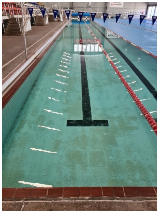
Figure 1: Image of 50m Pool Deterioration
