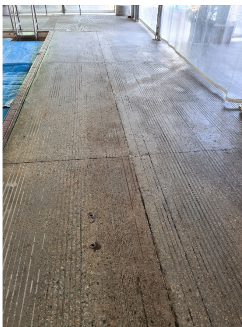
Figure 5: Image of Expansion Joints
