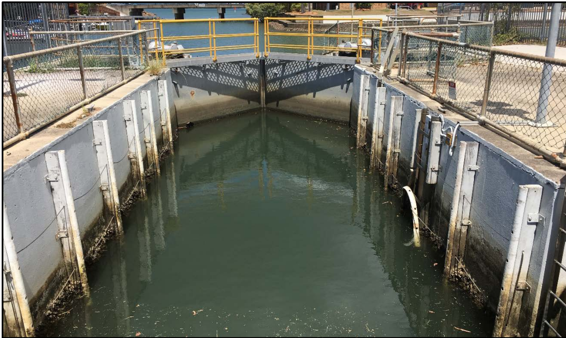
Figure 3 - View inside the lock bay, with lock gate and safety walkway in background
