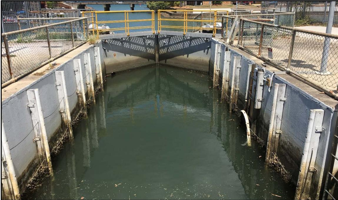
Figure 3 - View inside the lock bay, with lock gate and safety walkway in background
