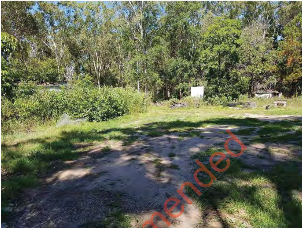
Photograph 1 – Existing site condition
