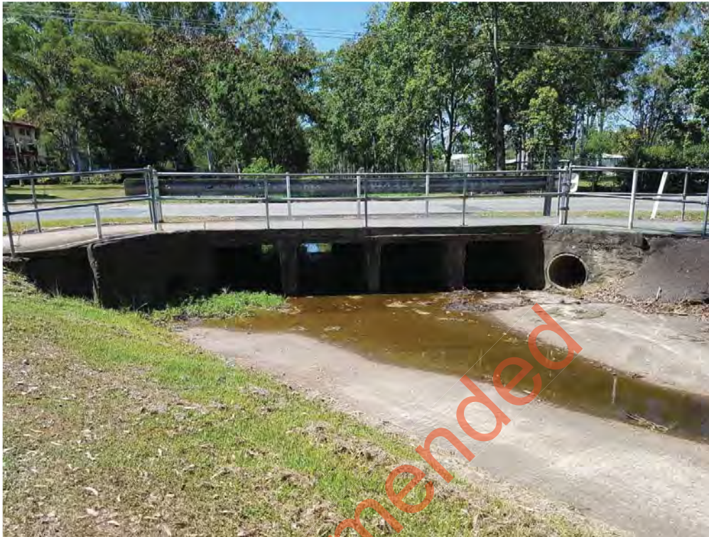
Photograph 3 – Culverts below Thompson Street
