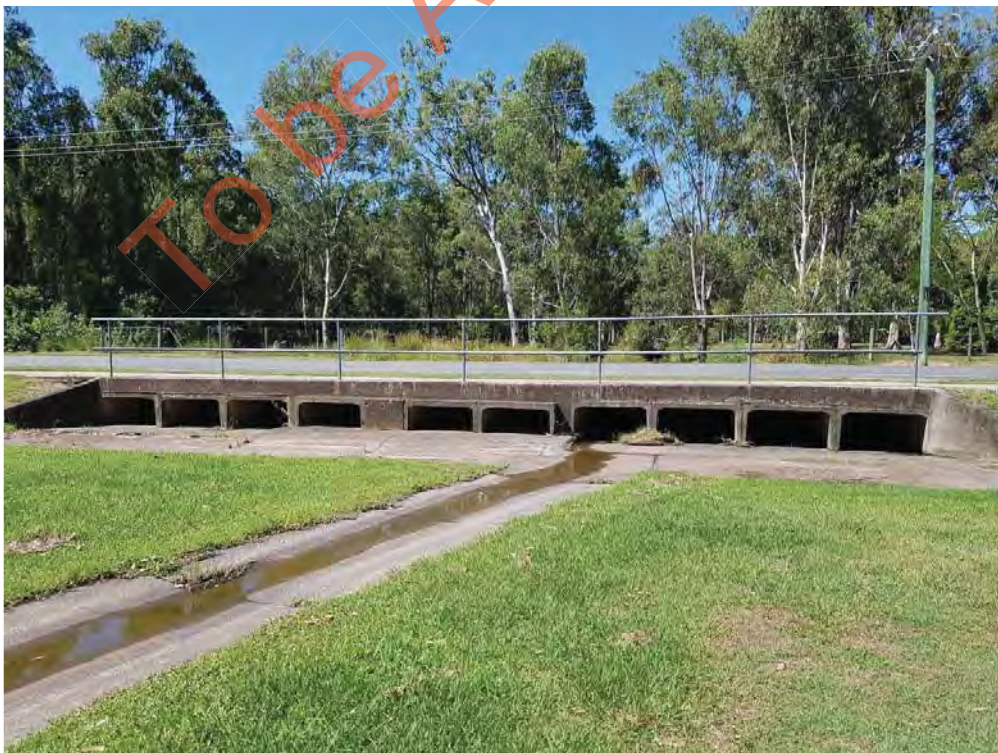
Photograph 4 – Culverts below Old Bay Road
