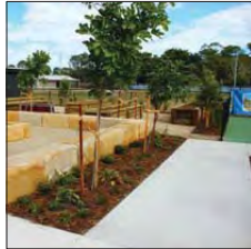
A GRADE SANDSTONE BLOCKS
