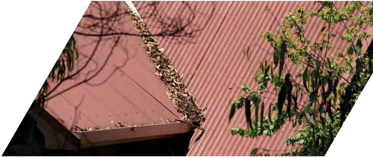
Complex house designs allow dead plant material and embers to accumulate.
