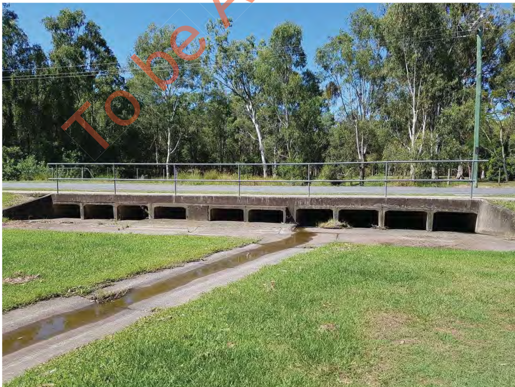
Photograph 4 – Culverts below Old Bay Road
