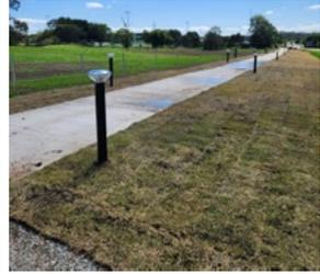
Installation of a 350 metre winding concrete pathway, 50 custom solar bollard lights, underground drainage, 78m of pedestrian safety fencing, removal and replacement of barbed wire fencing to adjacent horse paddocks, turfing and landscaping.
